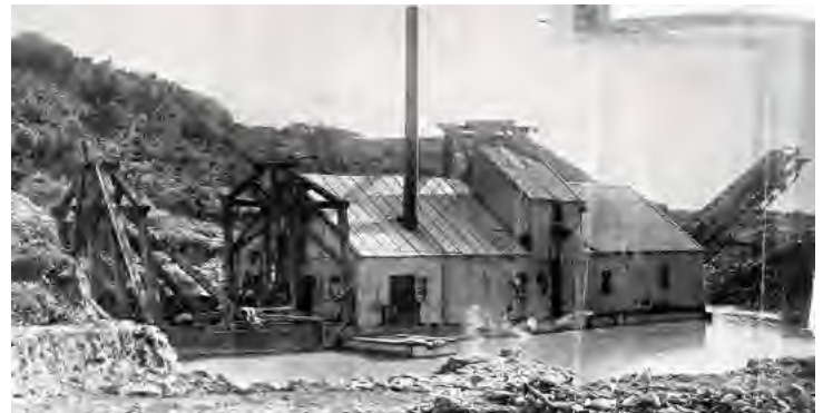
The largest steam-powered gold dredge in New Zealand at the time, was floated on the pond at Donoghues in 1902.
