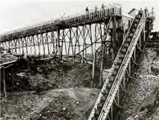
Impressive elevator plant on Donoghues
